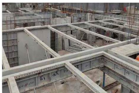
Assembling end beam panels
