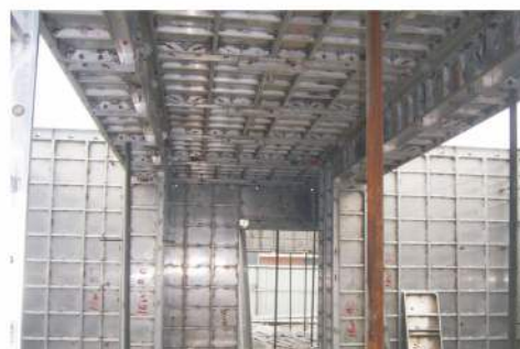
Assembling slab panels
