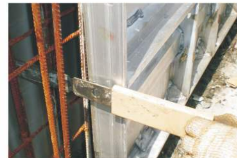
Assembling sleeve pipe
