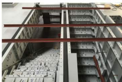
Assembling staircase
