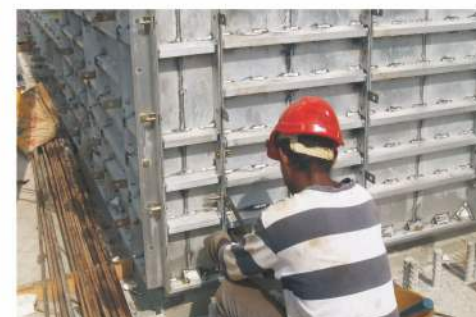
Assembling inner&outer wall panels
