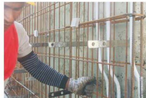
Assembling flat tie
