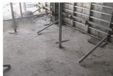
Reinforce the bottom
