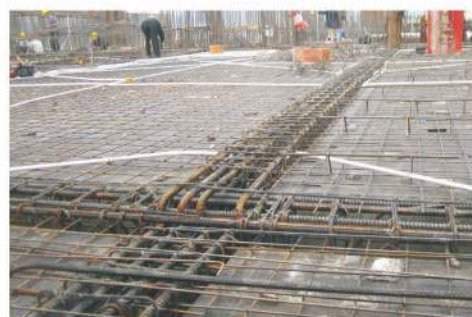
Binding rebars and assembling wire&pipes
